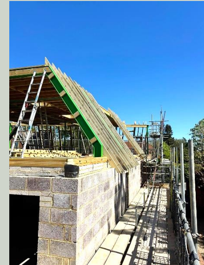
Good progress on Site 1...
